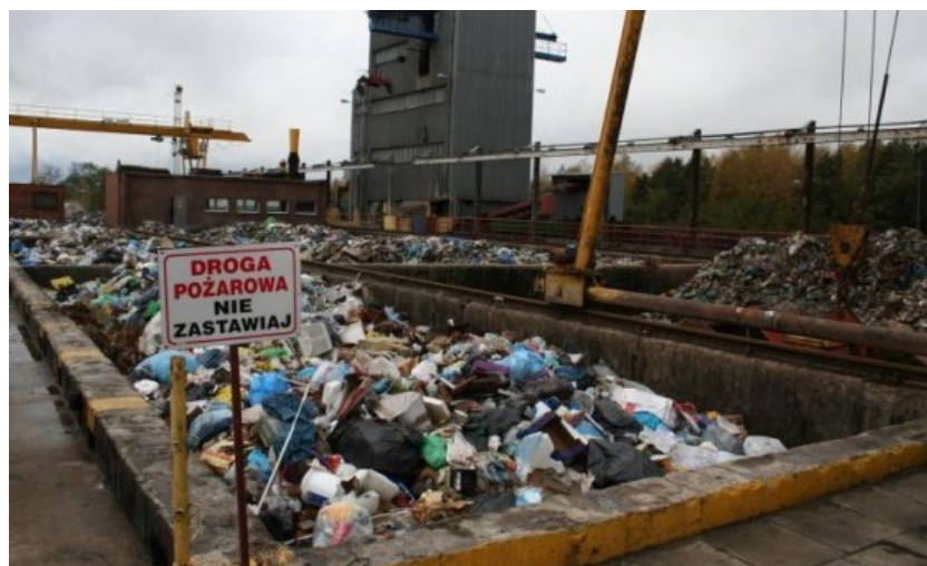
Figure 12: Waste Management Plant in Zielena Gora 198
